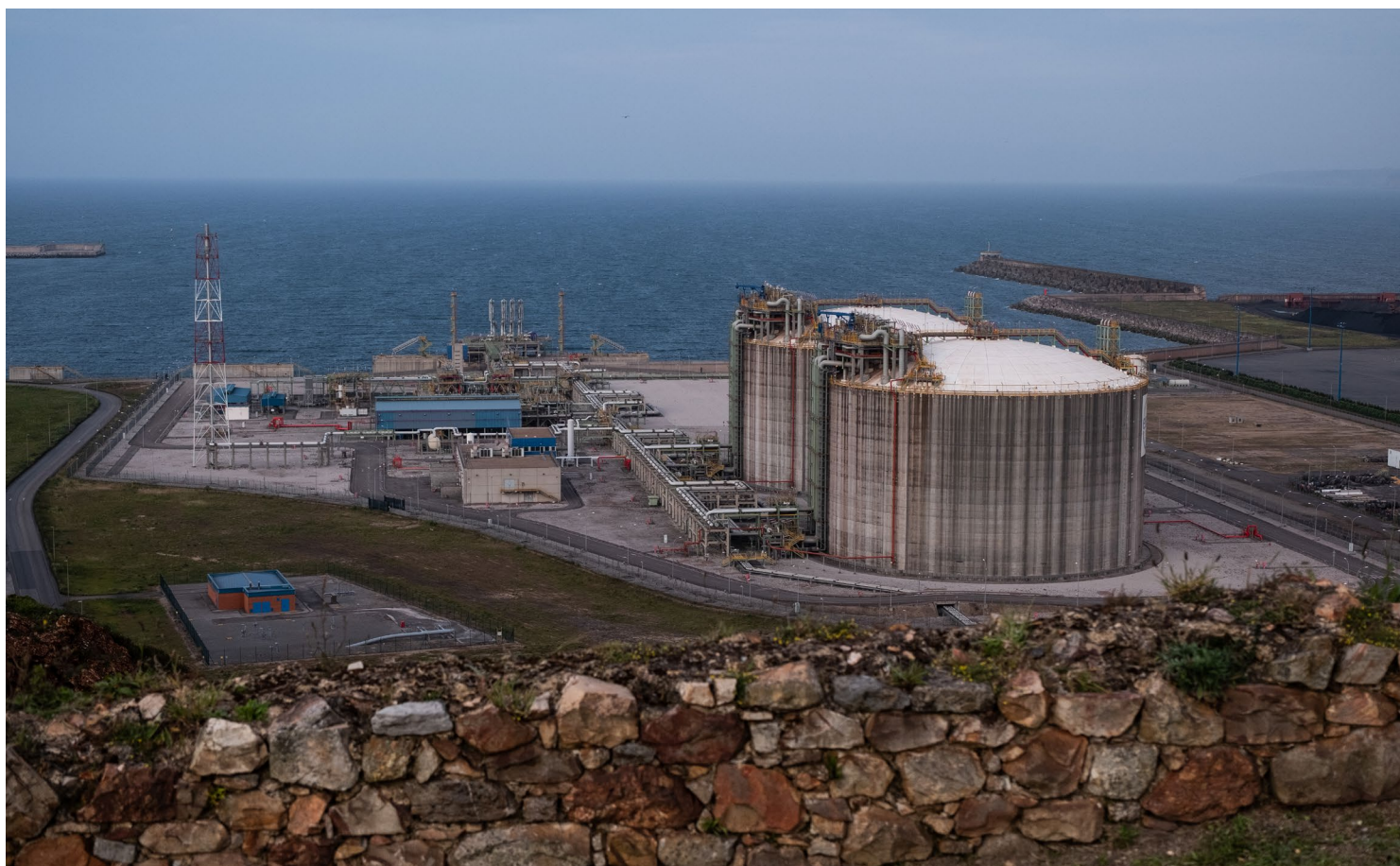
Regasification plant of El Musel in Gijón.
